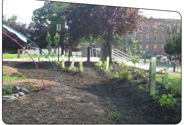
The Green Collar Futures team designed & installed a rainwater harvesting system that effectively doubles to triples the rainfall available to the garden, by diverting vast amounts of pavement-runoff into swales that feed the plants in the garden.
