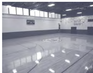
A view of the resurfaced basketball court floor and new roof at the North Camden Community Center Gym.
