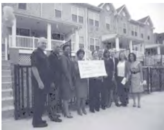
Mayor Redd and representatives from Saint Joseph's Carpenter Society, Wells Fargo Regional Foundation and Cooper's Ferry Partnership standing in front of the newly constructed homes in East Camden.
